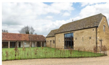
Barn at Arms Farm - recently converted to residential use. Late C18, rubble stone with stone slate half-hipped roof - south side hipped projecting cart-entry
