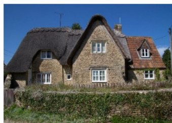
62/64 High Street - C17, rubble stone with thatched roof with later extension
