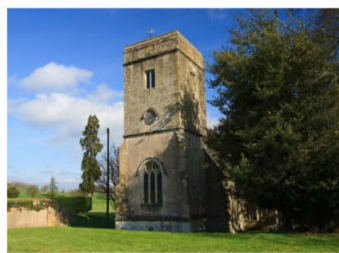
Church of St James - Draycot Cerne Grade II* - c1300 with C16 west tower, altered in mid C19, rubble stone, ashlar tower, stone slate roof
