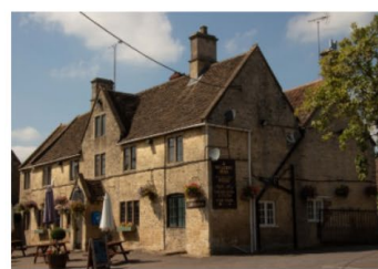
Wellesley Arms Public House - mid C18, rubble stone with stone slate roof
