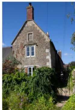
68/70 High Street - Pair of houses, C18, roughcast rubble stone with pantiled roof
