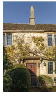
Ross Cottage dates from 1782 - rubble stone with stone slate roof
