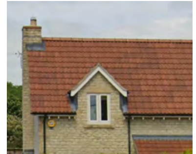
Careful consideration should be given to high quality materials and the level of detailing to add interest brightly coloured tiles should only be made of clay, where they will dull over time
