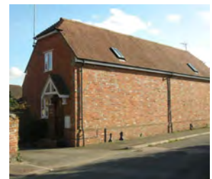
Domestic style porch and windows often alters the barn character to a more residential and confused appearance
