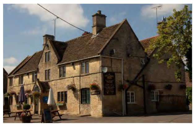
Wellesley Arms Public House - mid C18, rubble stone with stone slate roof,
